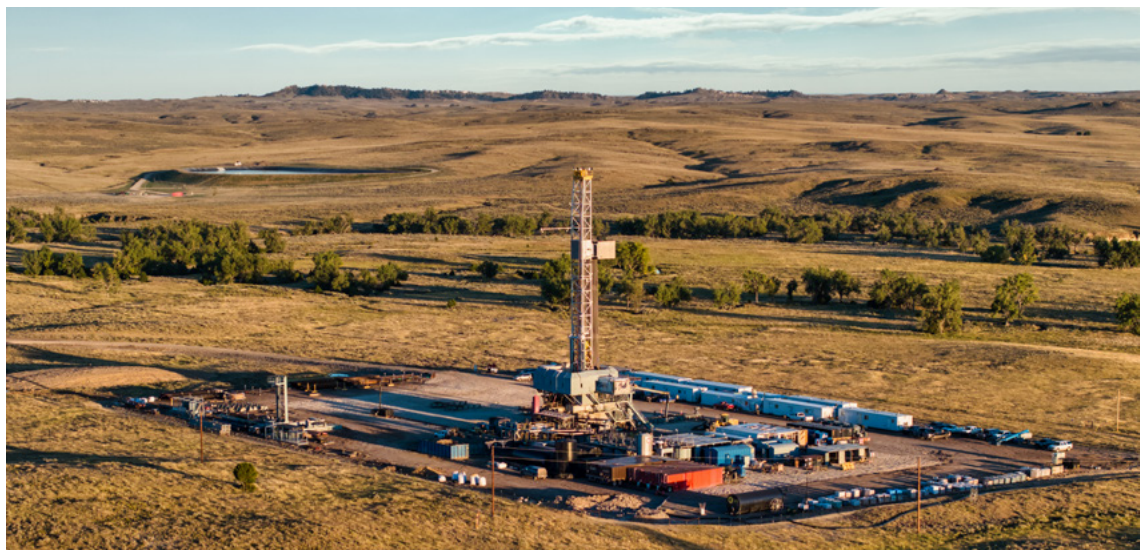
1876 RESOURCES WELL ON THE NETZ PAD, WYOMING
